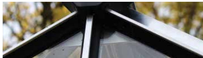
Toughened glass with capping
